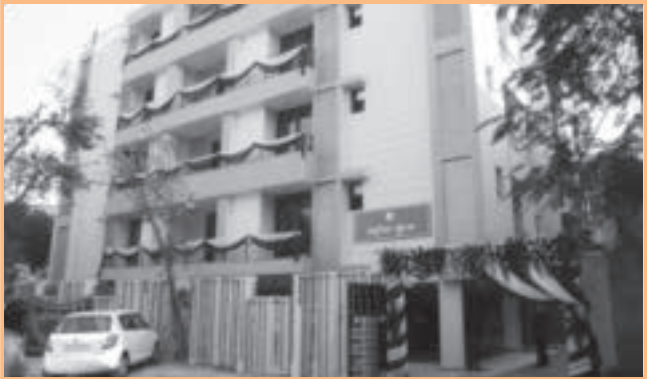
New residential premises at East of Kailash, New Delhi.
