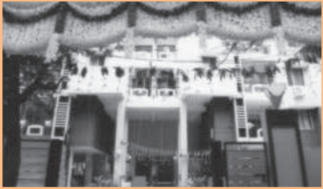
New Premises at Cenotaph Road, Chennai
